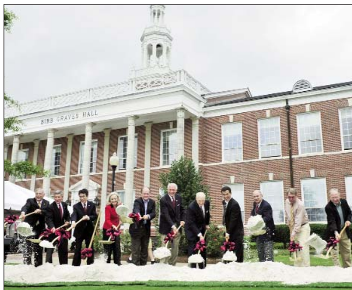
Officially breaking ground on Troy University's renovation and addition to Bibb Graves Hall are (left to right) Alabama Development Office Director Neal Wade; Senior Vice Chancellor for Advancement and External Relations Dr. John Schmidt; Consul of Education Zhou Haibao, Confucius Institute; Sorrell College of Business Interim Dean Dr. Kaye Sheridan; Congressman Bobby Bright; Chancellor Jack Hawkins, Jr.; Executive Vice Chancellor and Provost Dr. Ed Roach; Director and Consul of Education, Dr. Yan Guohua, Consulate General People's Republic of China (Houston, Texas); Troy University Board of Trustees member Charles Nailen; architect Walter McKee; and general contractor Clyde Bear.
