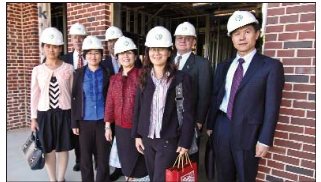
Members of the Confucius Institute’s Board of Directors take a tour of ongoing renovation work at Bibb Graves Hall.
